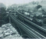
Millers Dale Station E.R. Morten
