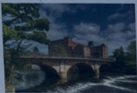
Belper Mills and River Bridge Ashley Franklin
